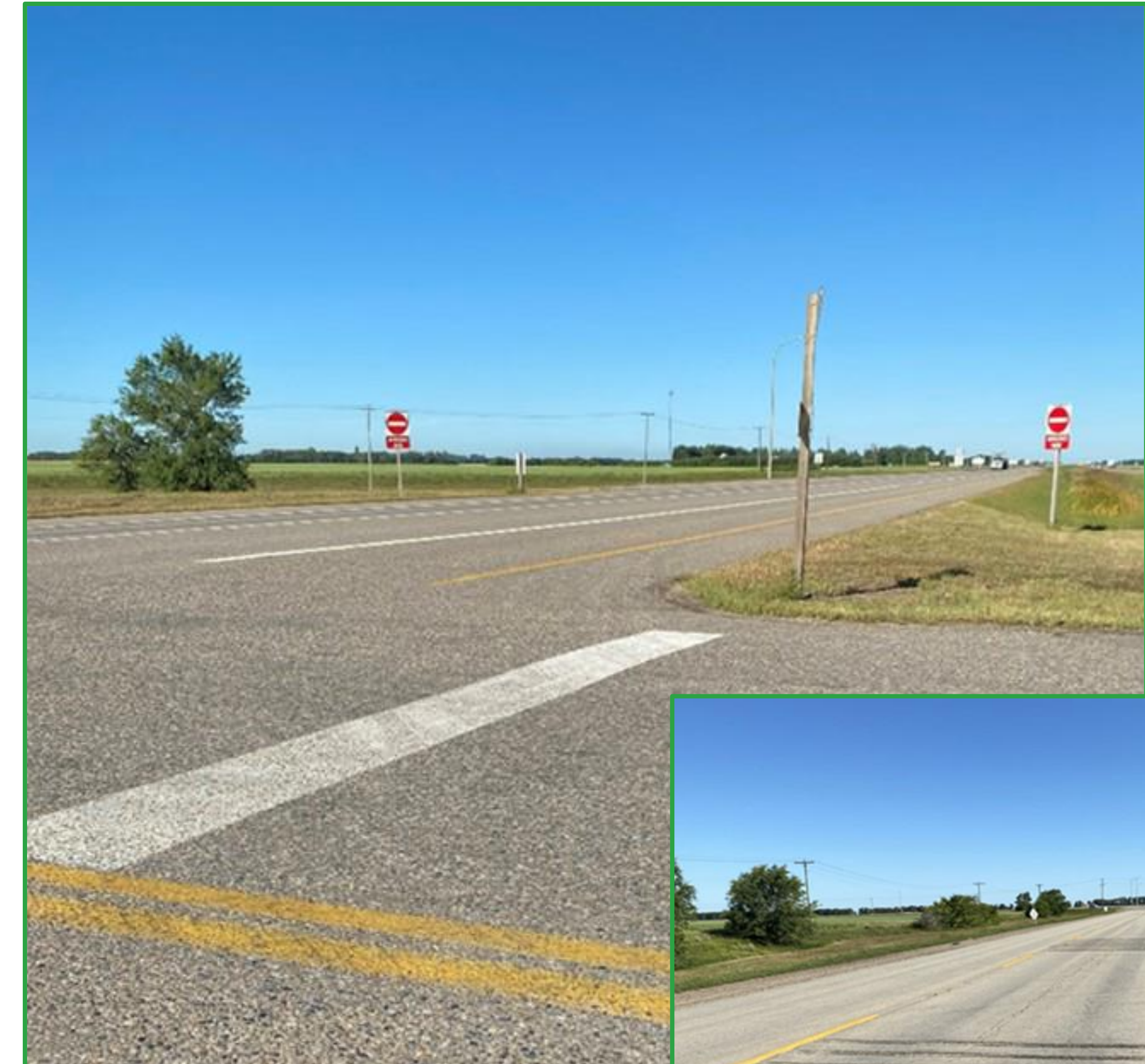
Refurbished pavement markings at the intersection.
