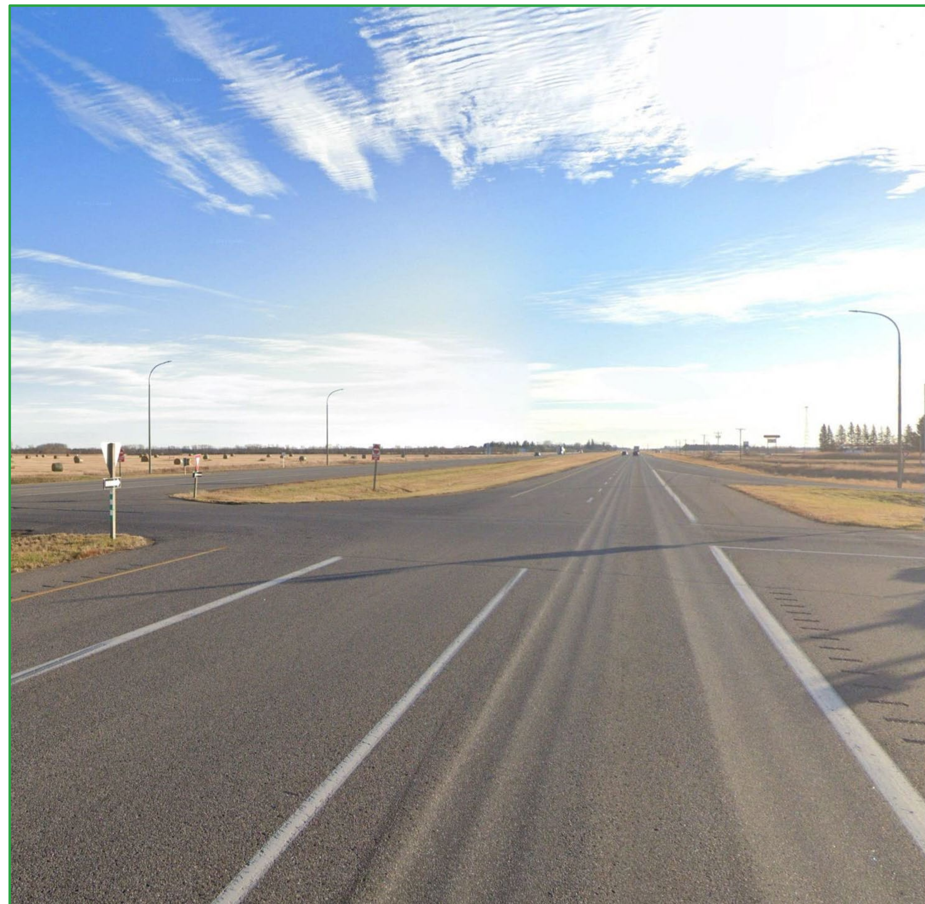
PTH 1 and PTH 5 intersection looking east.
